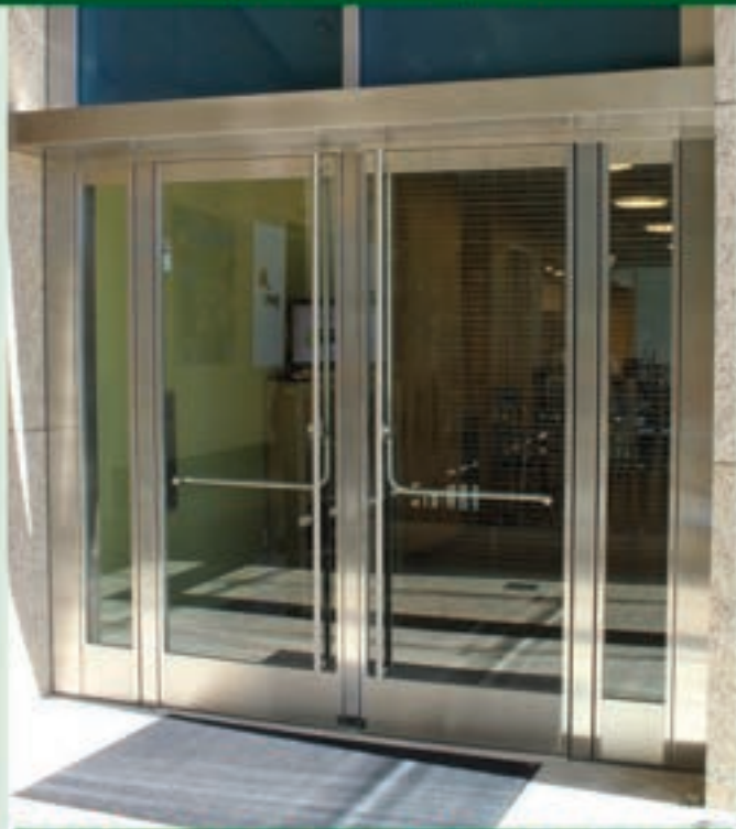
Full Frame Cladged Doors with Round Bar Panic Device
